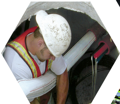
Outside Plant/ GPON/EPON/ RFoG
